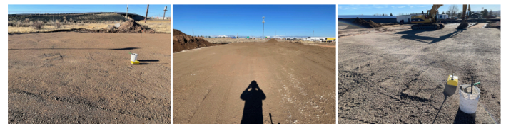
Southeast parking lot
